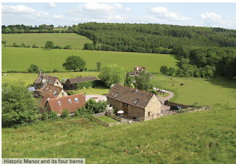
Historic Manor and its four barns
