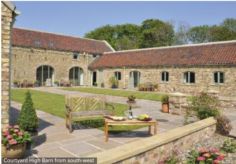
Courtyard High Barn from south-west
