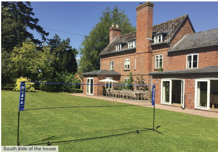
South side of the house
